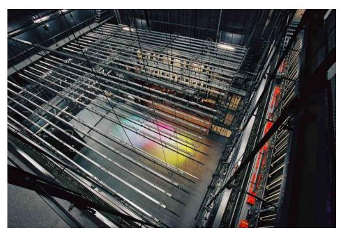
Being a light weight 50mm bar with ample loading capacity, the K31 is also widely used to as part of theatre fly system.
